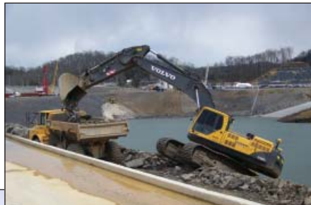
TOP: A hydraulic backhoe loads rock and rubble into a dump truck.
