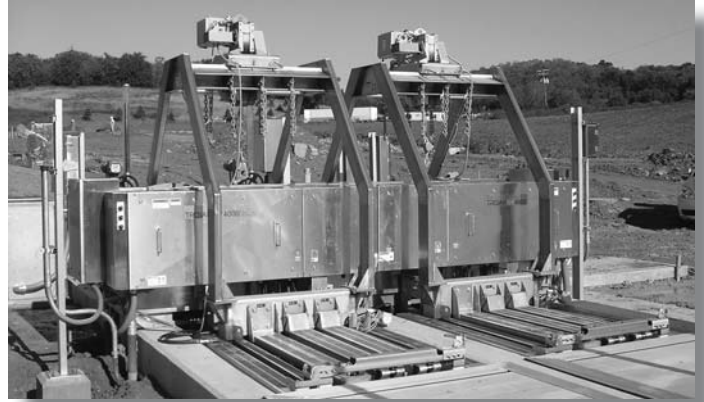
The treatment facility uses state-of-the-art disinfection with ultraviolet light and biofiltration technology for odor issues. Photo by Sanitation District No. 1
