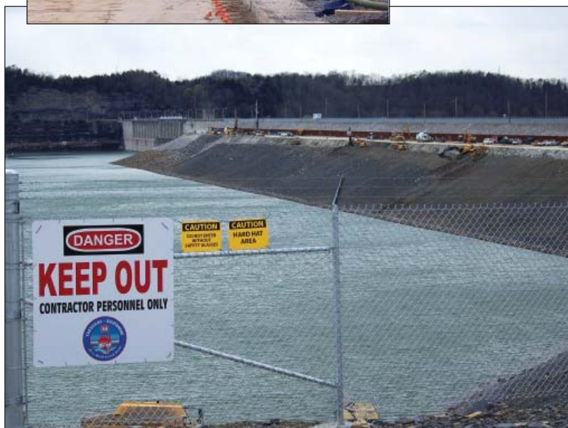
BELOW: Contractors from Italy and France have begun construction of a massive concrete wall embedded deep within the earthen portion of the dam.
